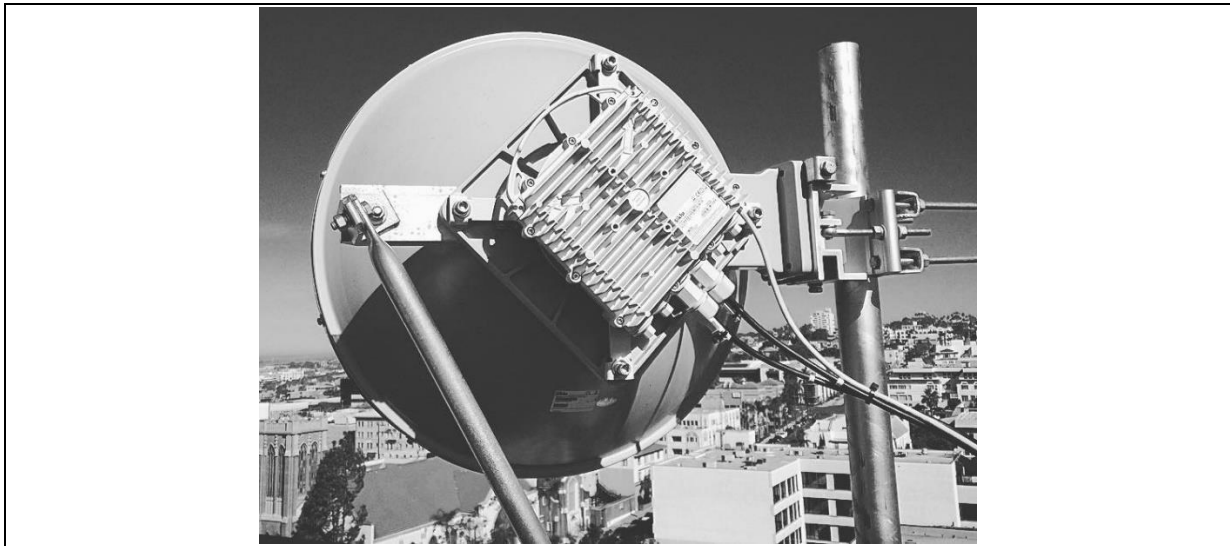
FIGURE 4a: 2FT Antenna installation (EH-ANT-2ft-B)
